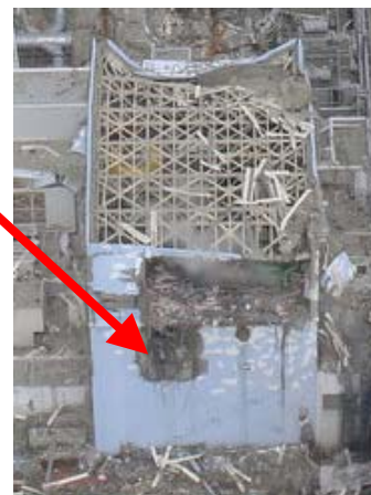
Figure Photo of F4 on March 20th.
