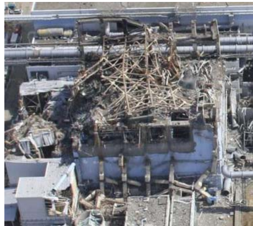
Top (5th) floor and walls at 4th floor were destroyed.
