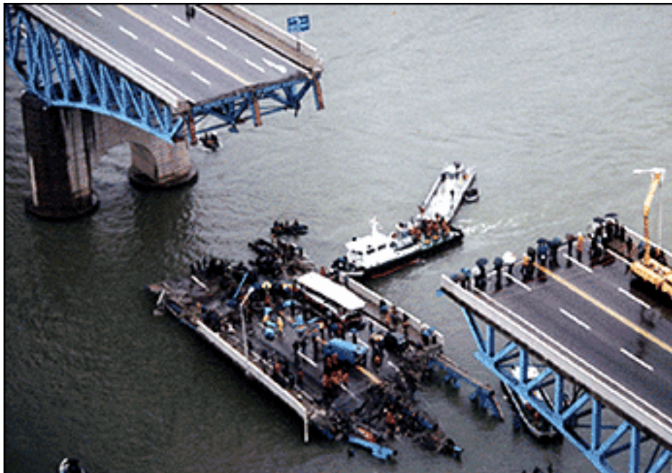
Photo.-1. the situation right after the decay falling accident of Seongsu Bridge. (Donation: Prof.Yozo Fujino, University of Tokyo)
