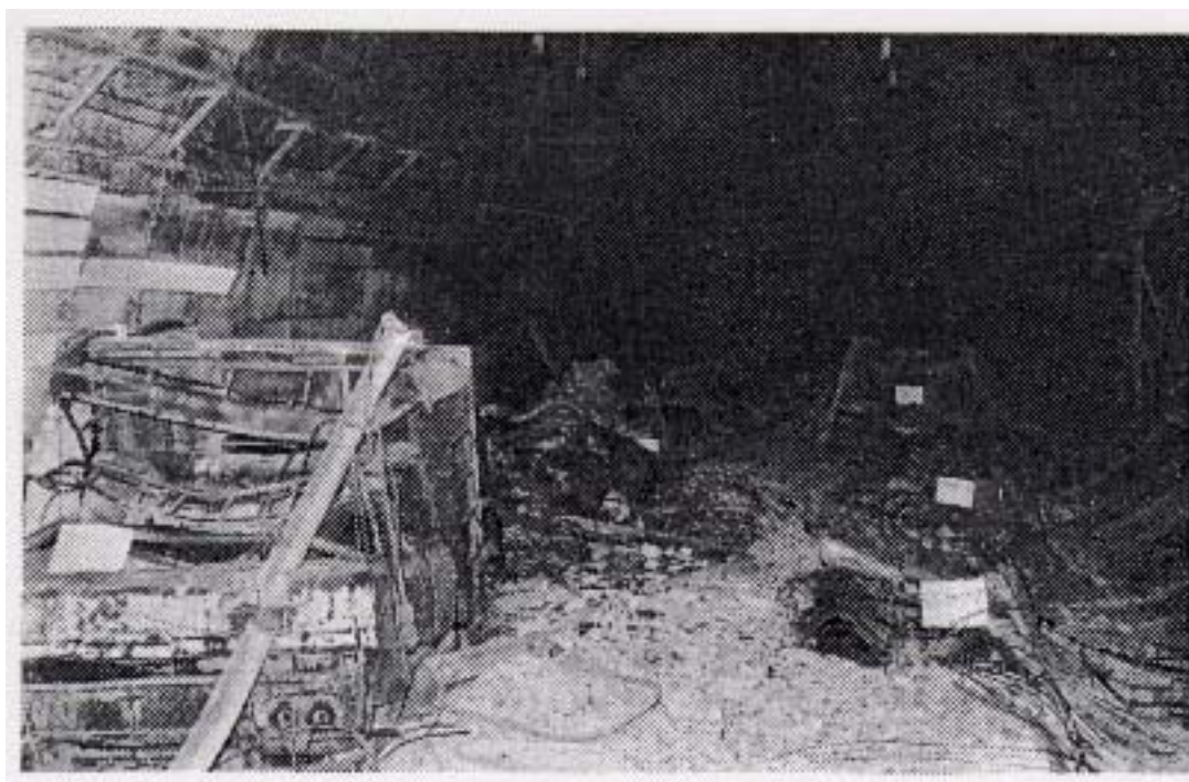
Picture 1 The condition 1240m from the Shizuoka-side Exit (Source: Highway and car. The research community of highways, Nihon-zaka tunnel's fire disaster and its aid actions)
