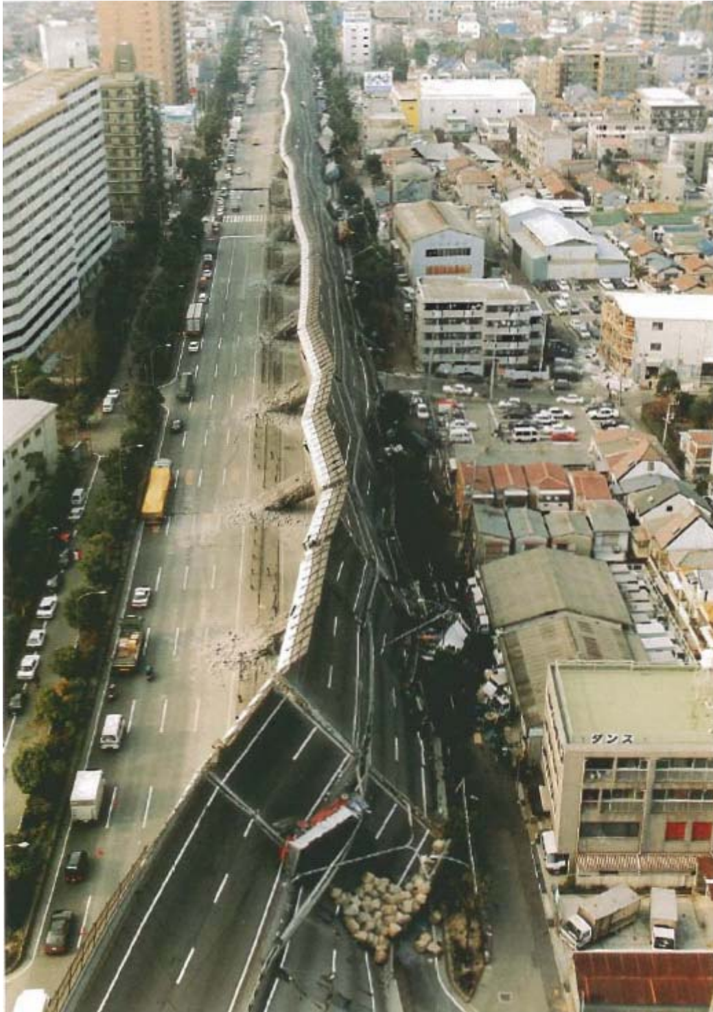
Figure 3 Collapse of the Pilz elevated bridge of Hanshin Expressway Kobe Line
