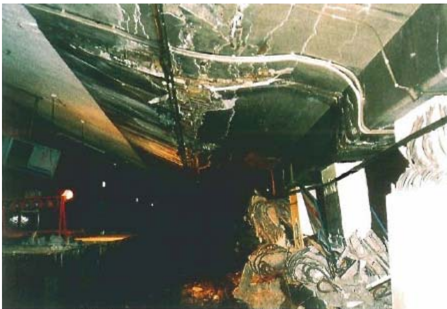
Figure 5 Crushing of the central pillar of Daikai Station of Kobe Express Railway and collapse of the upper floor panel (Source: Architectural Institute of Japan, Picture: Prof. Iwadate)
