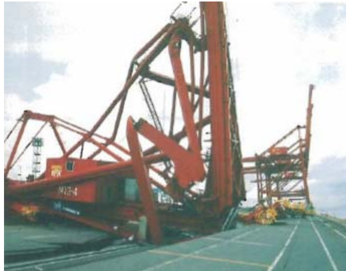
Figure 6: Collapse of the RC3-4 crane at Rokko Island (Only one crane totally collapsed.) (Source: Japan Society of Civil Engineers)
