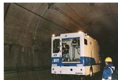
Figure 5. Inspection by SATUZO (Source: West Japan Railway Co)
