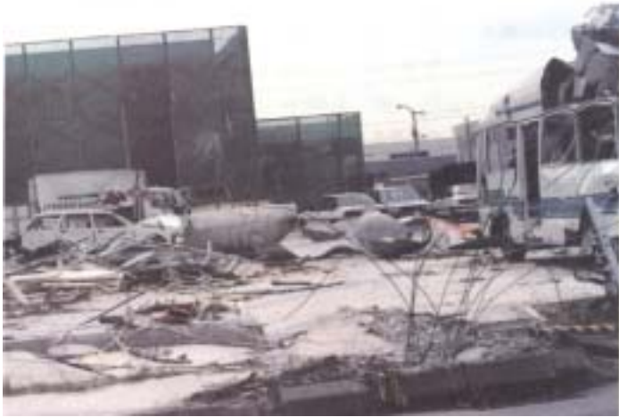
Fig. 4 Appearance of damage (Part 3).
