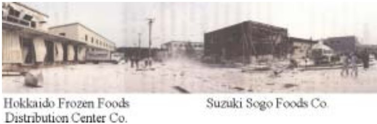
Fig. 2 Appearance of damage (Part 1).
