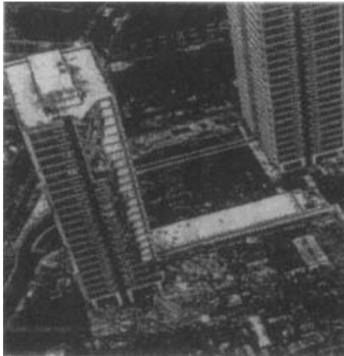
Photo 1. Collapsed 22-Story Southeast Corner [1]
